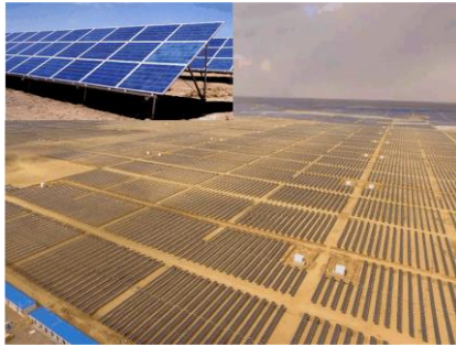
Fig. 3. PV plant experimental prototype.
